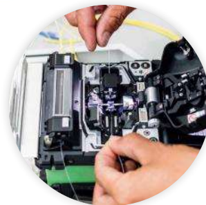
FIBER OPTIC EQUIPMENT
